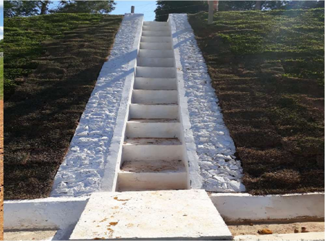
Figura 5.6 – DCD. Pedra argamassada
